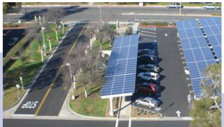
City Hall ADA and Visitor Parking with 10% Solar Panel Array Visible
