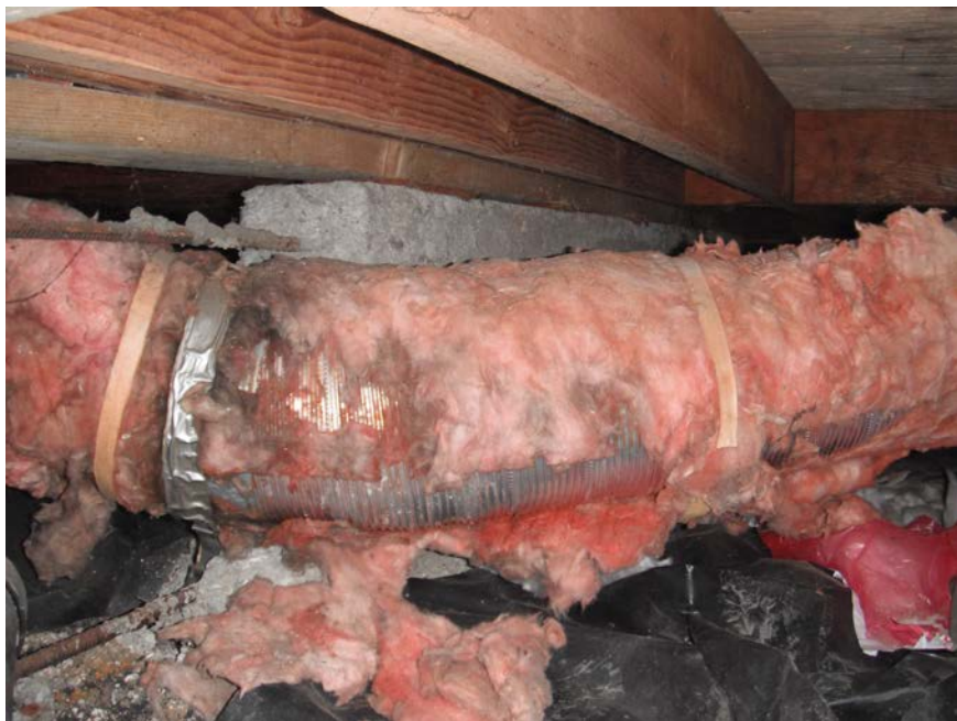
Poor insulation
