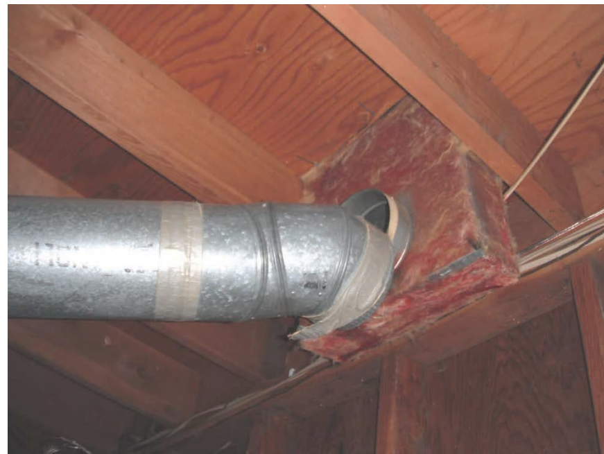
Disconnected ducts
