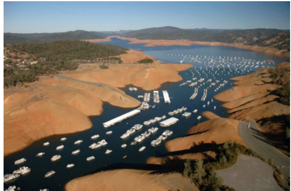
Oroville Reservoir, January 2014
