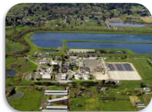
Waste Water Treatment Plant
