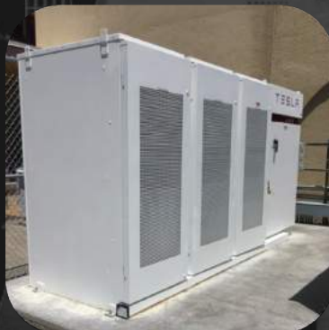
335 kW / 669 kWh Battery System Pleasanton, CA
