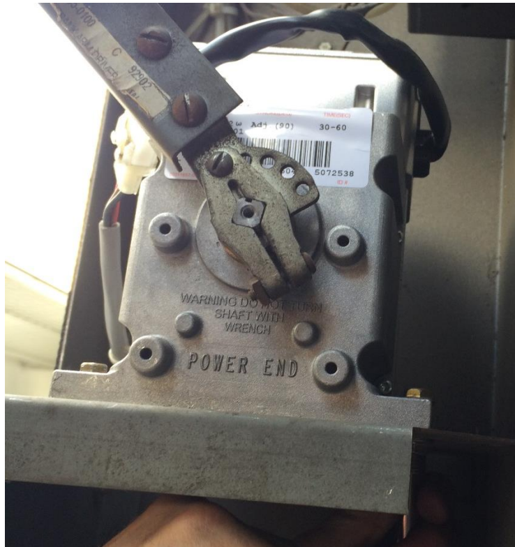
Figure 3.4: New Actuator Installed
