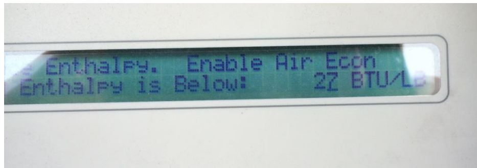
Figure 3.5: New Enthalpy Set point at 27 Btu / lb
