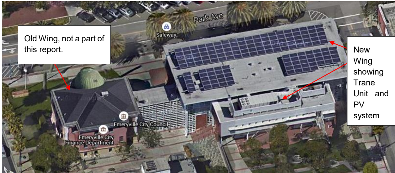
Figure 2.2: Satellite view of Emeryville Civic Center
