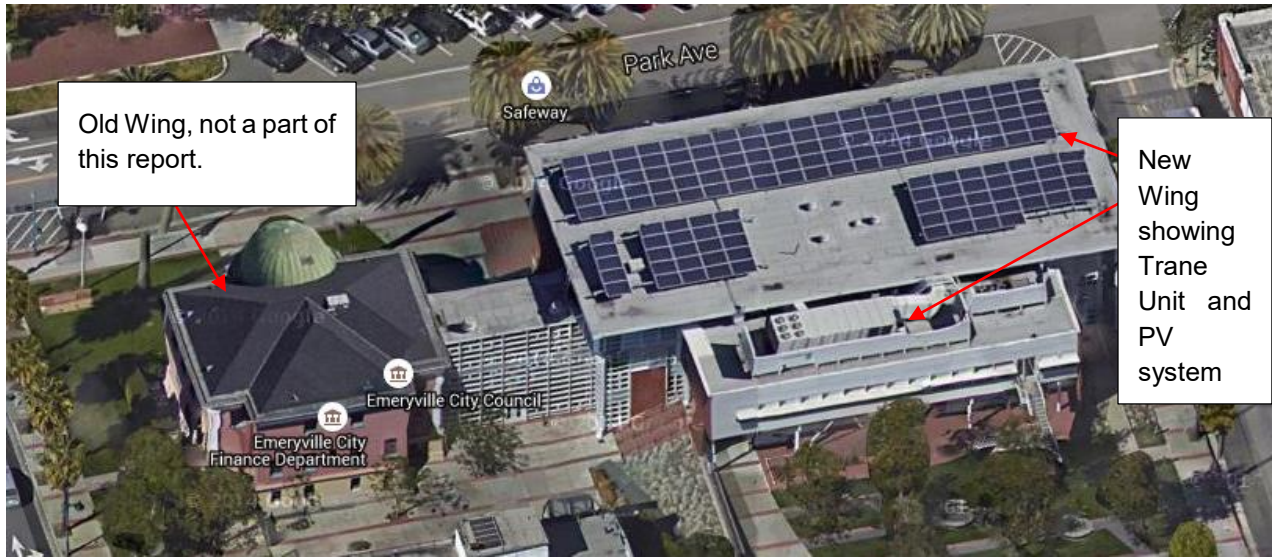
Figure 2.2: Satellite view of Emeryville Civic Center
