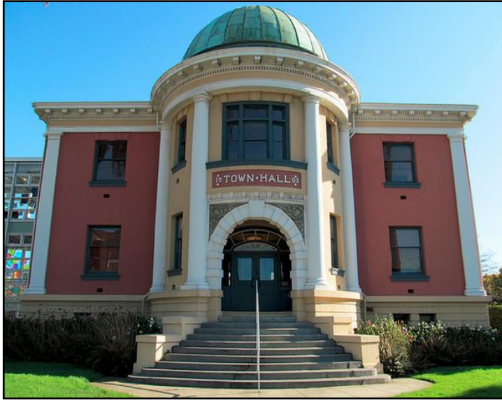
City of Emeryville, Town Hall
