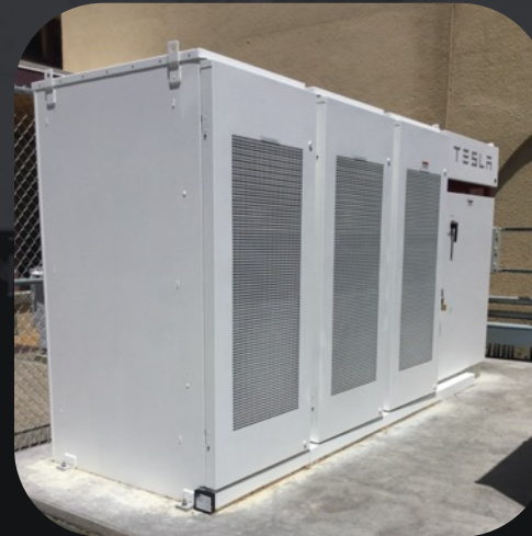
335 kW / 669 kWh Battery System Pleasanton, CA
