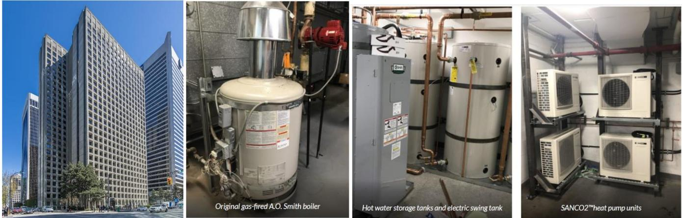
Figure 18: Arthur Erickson Place (left)<sup>52</sup>, the original gas-fired hot water boiler (center left), and the electrified heat pump water heater plant storage tanks (center right) and CO<sub>2</sub> heat pumps (right).
