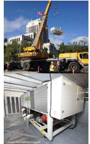
**Figure 11: Vancouver city hall and the Aermec 4-pipe heat pump installed and being installed with a crane.**
