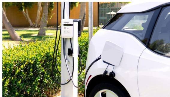
Level 2 240V 10-25 miles charged per hour
