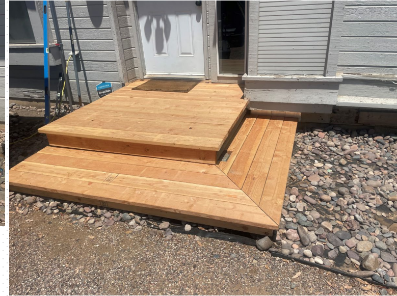
New Deck and Porch built with Treated Lumber
