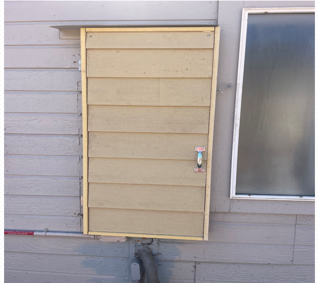
New Crawl Space and Electrical Panel Door built from non-combustible Hardie Board
