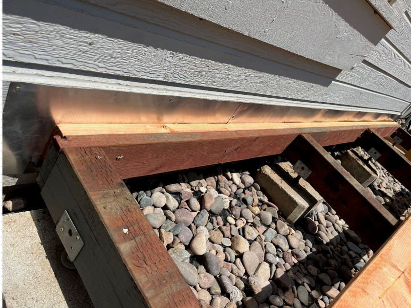
Metal Flashing where the deck meets the wall
