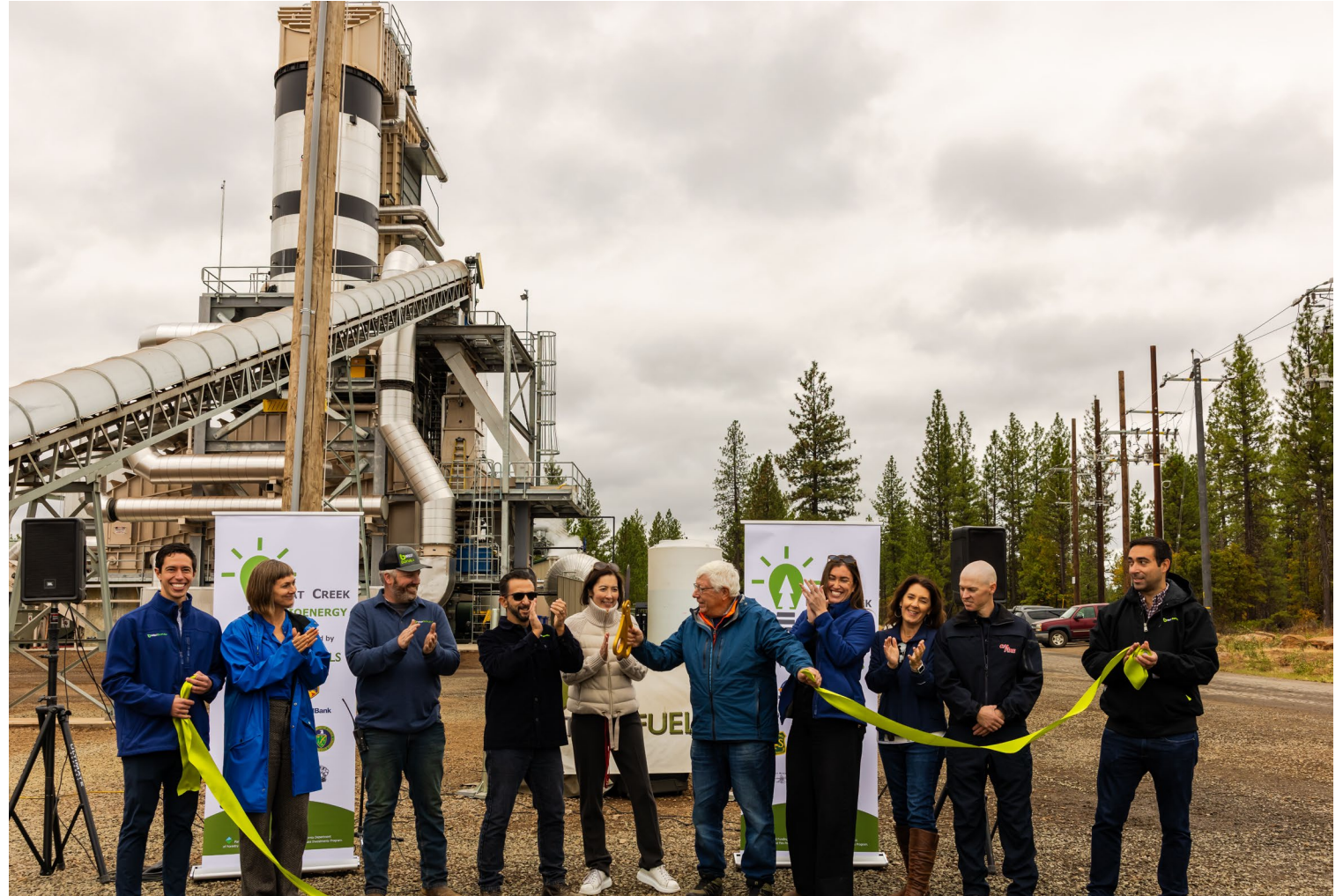
Figure 3: Burney-Hat Creek Bioenergy, LLC began commercial operations of this forest biomass bioenergy facility located in Shasta County (Source: CEC)
